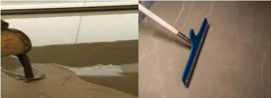
(2) Put on spiked shoes and enter the pouring area, use the air release roller to roll gently to eliminate the bubbles generated during mixing, pouring and pouring.
