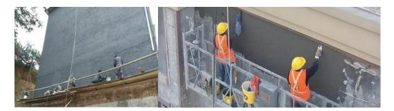
□In waterproof and impermeable projects with special requirements, after the waterproof mortar is dry, one or two coats of HQG-4<sup>#</sup> huaqianjiao can be sprayed "wet to wet" for surface treatment, further enhancing the waterproof effect. This not only prevents negligence and omissions during the construction of waterproof
