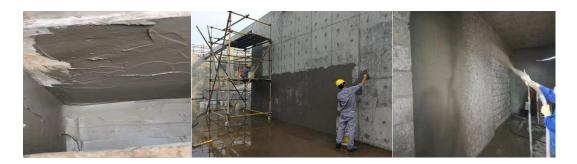
Dayered construction: The recommended thickness for a single construction is no more than 2mm. After the initial setting of the first layer (usually around 4 hours for initial setting and 8 hours for final setting), the second layer should be applied until the design thickness is reached. The construction direction of the front and back should cross to avoid missed brushing, scraping, and plastering.
